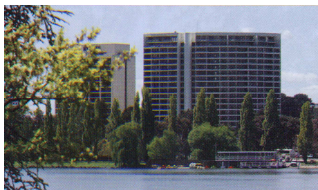
Fot. 3. Pacific International Apartments (Canberra, Australia)
