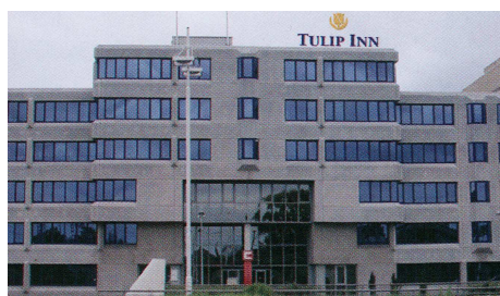
Fot. 6. Tulip Inn Leiden Centre (Lejda, Holandia)
