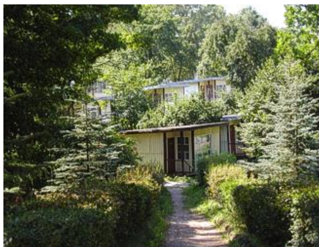
Fot. 6. Zniszczony park w Cieszynie Drawskim (fot. autor) Photo 6. Devastated park at Cieszyn Drawski (photo author)
