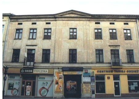
Fot. 2. Hotel Metropol – stan obecny (autor) / Metropol Hotel – nowadays (author)
