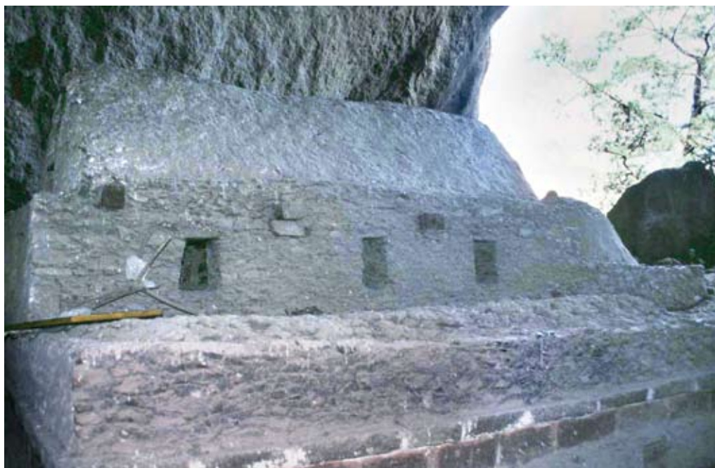
5. ʿMākina Mādhane Alām church, superstructure, south side
