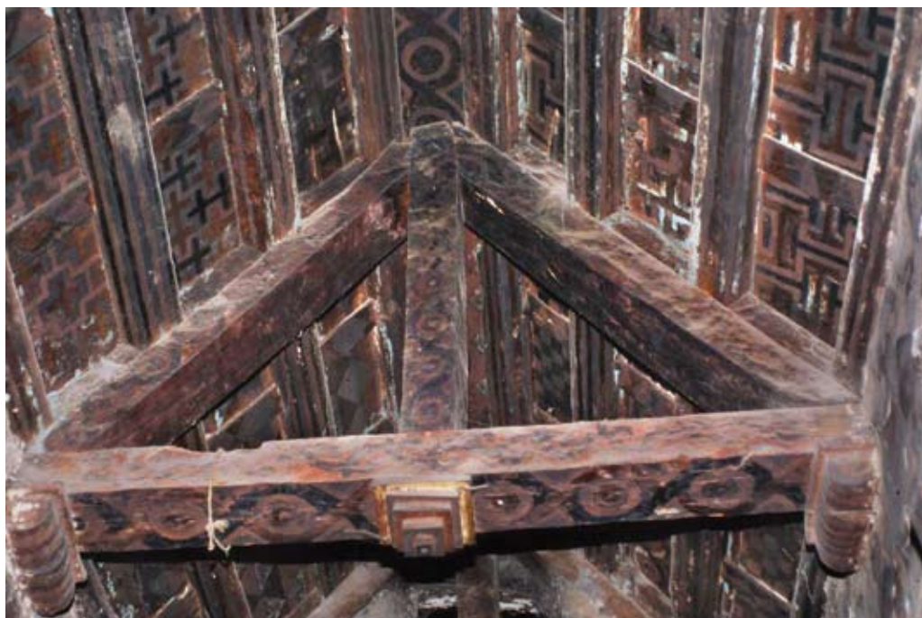
13. ፻mäkina Mädhane Aläm church, kingpost, tie beam and principal rafters supporting saddle-back roof
