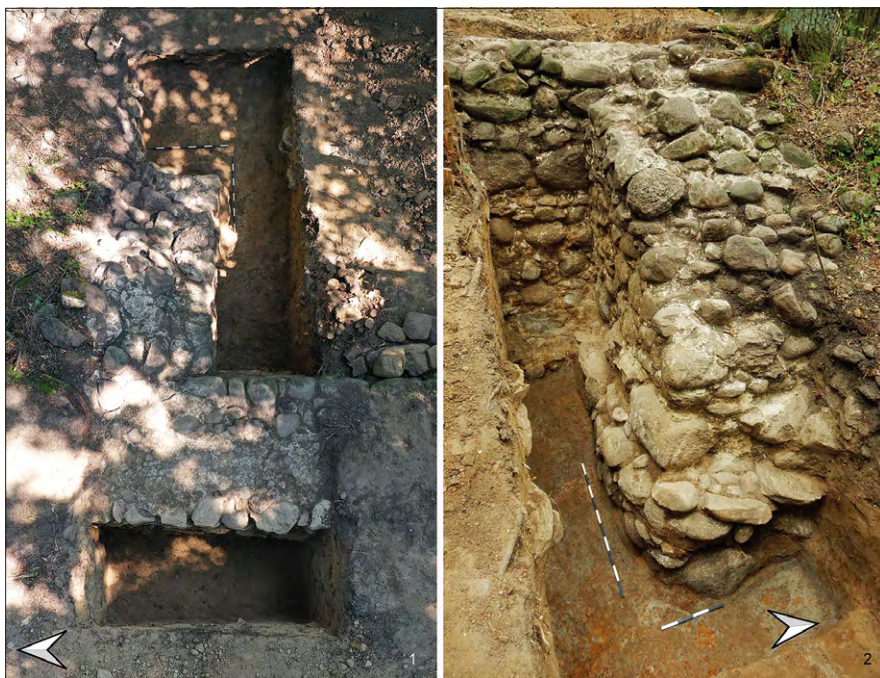
Fig. 9. Remains of the foundation wall with adjacent avant-corps. Outline (1) and section (2). Photo: Hubert Augustyniak.
