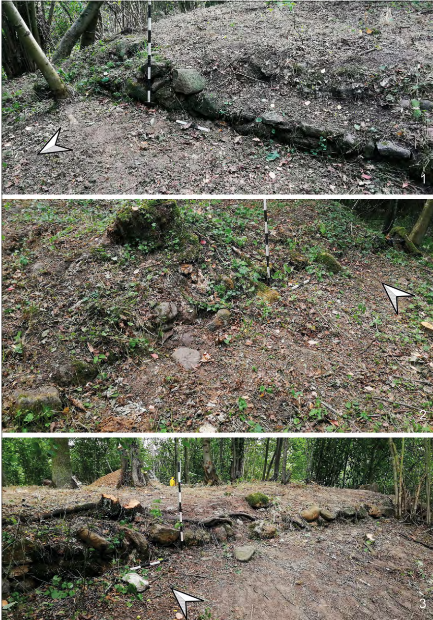
Fig. 8. Remains of the outer wall visible in the north (1), west (2) and southern part of the seat. Photo: Arkadiusz Michalak.
