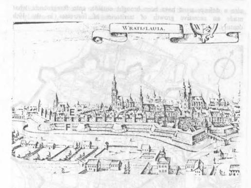
Fig. 6. Wrocław (Breslau), Acc. to: M. Merian, Topographia Bohemiae, Moraviae et Silesiae..., Franckfurt 1650. E - the medieval defensive wall with turrets, F - the modern (16th century) rampart with bulwarks and bastions
